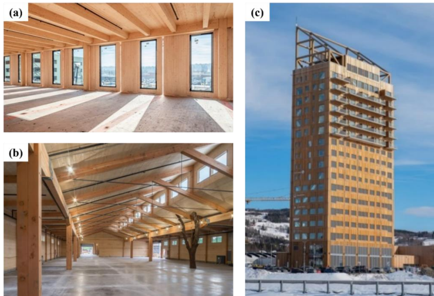
Figure 10. (a, b) Cross-laminated timber usage areas (URL-9); (c) Mjøstårnet building in Norway (URL-10).
